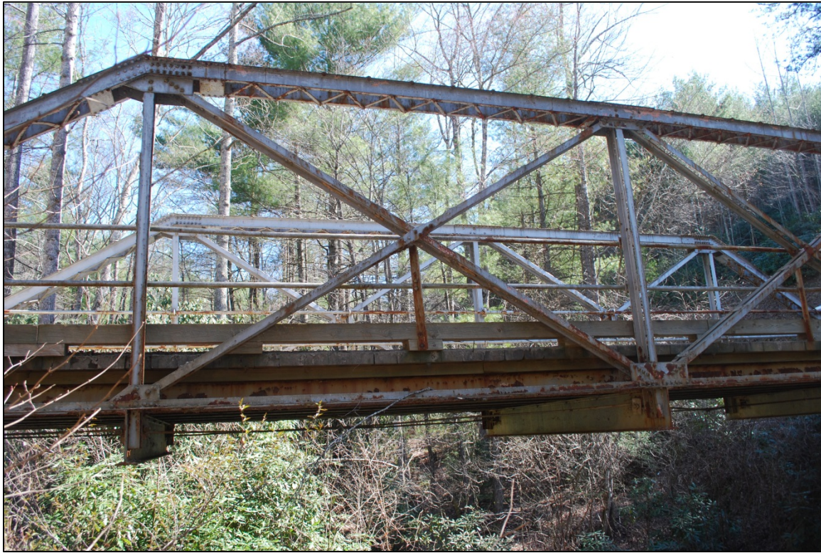
Figure 8: South elevation looking north.
