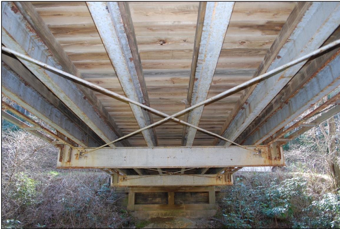
Figure 9: View of substructure of Bridge No. 110.
