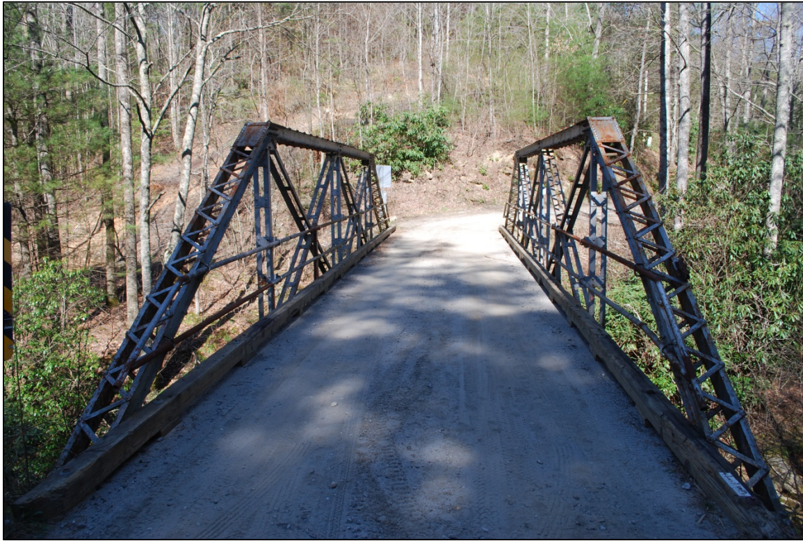
Figure 6: Bridge No. 110, looking northwest on SR 1363 (Walsh Road).
