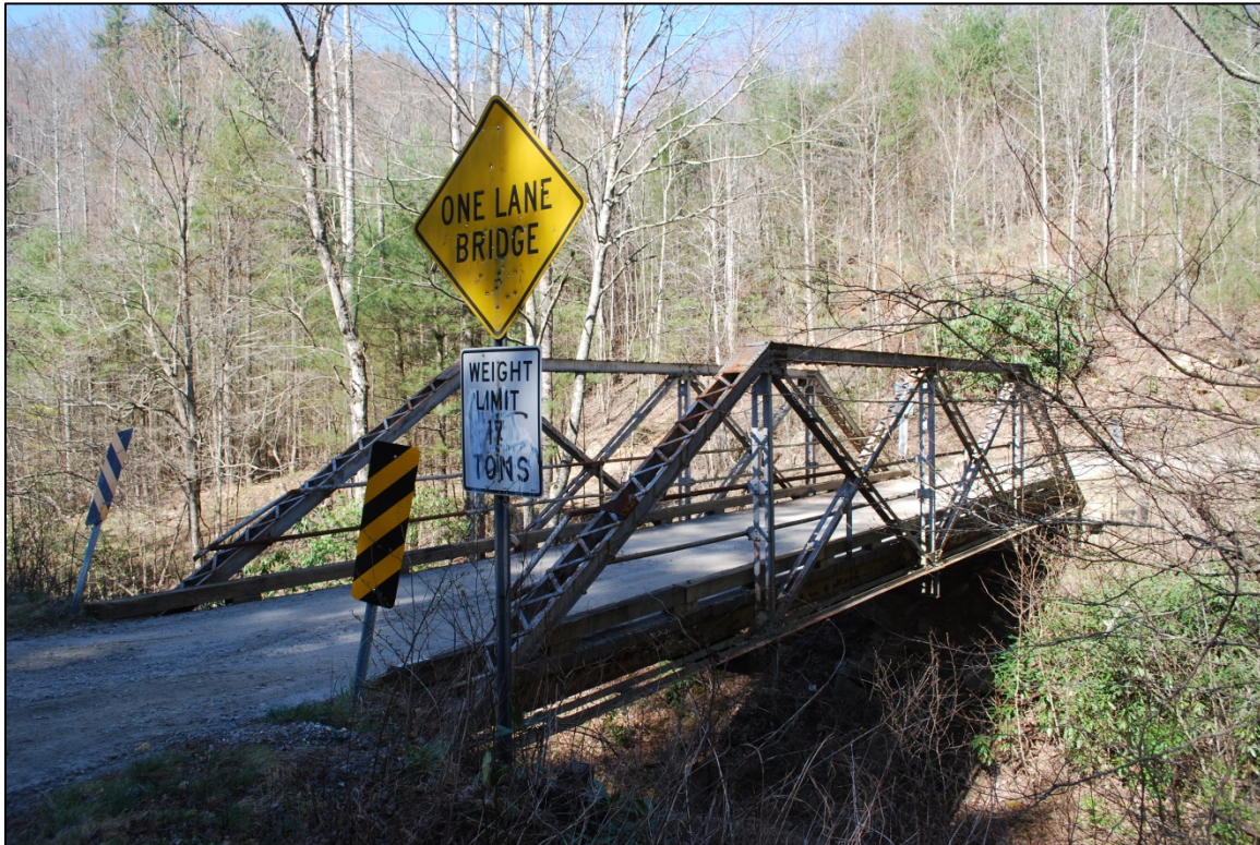
Figure 3: Bridge No. 110, looking southwest.
