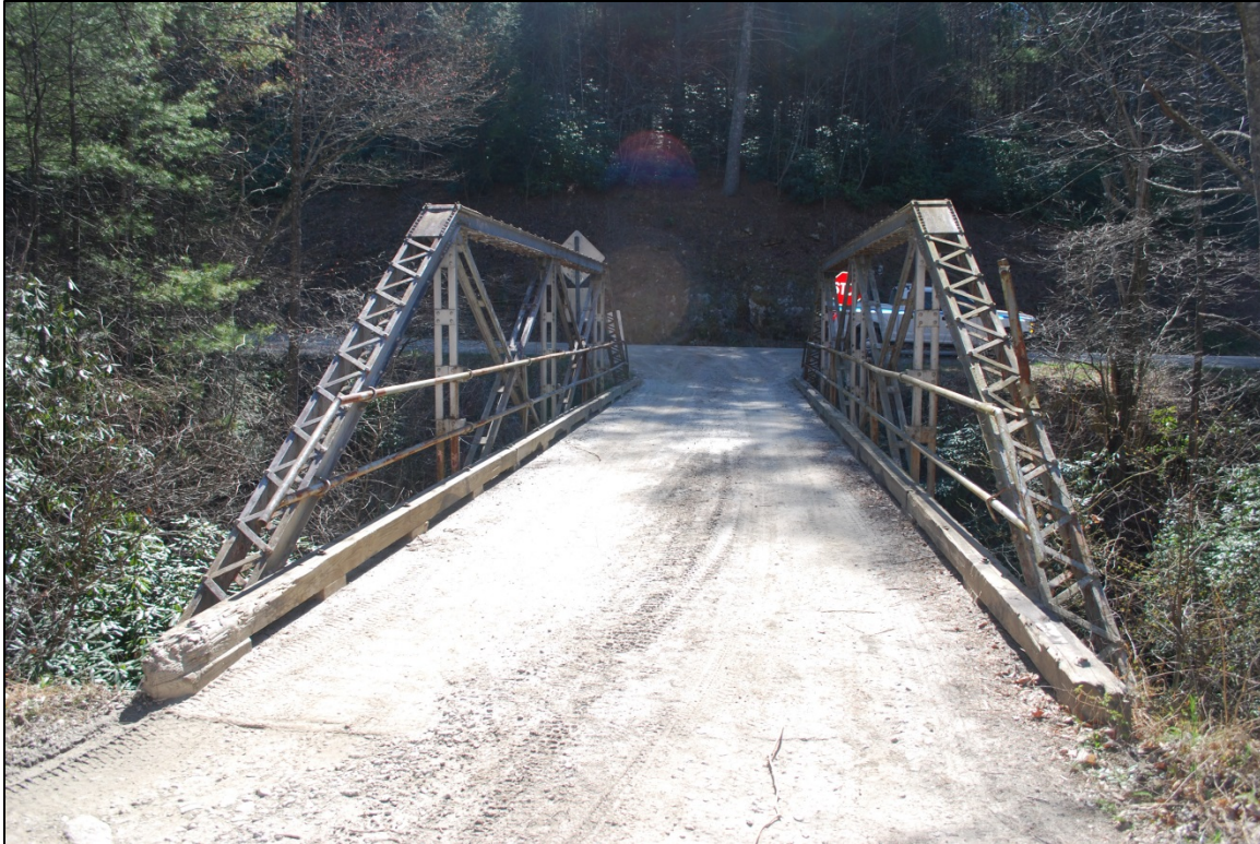
Figure 5: Bridge No. 110, looking southeast towards SR 1362 (Big Ivy Road).
