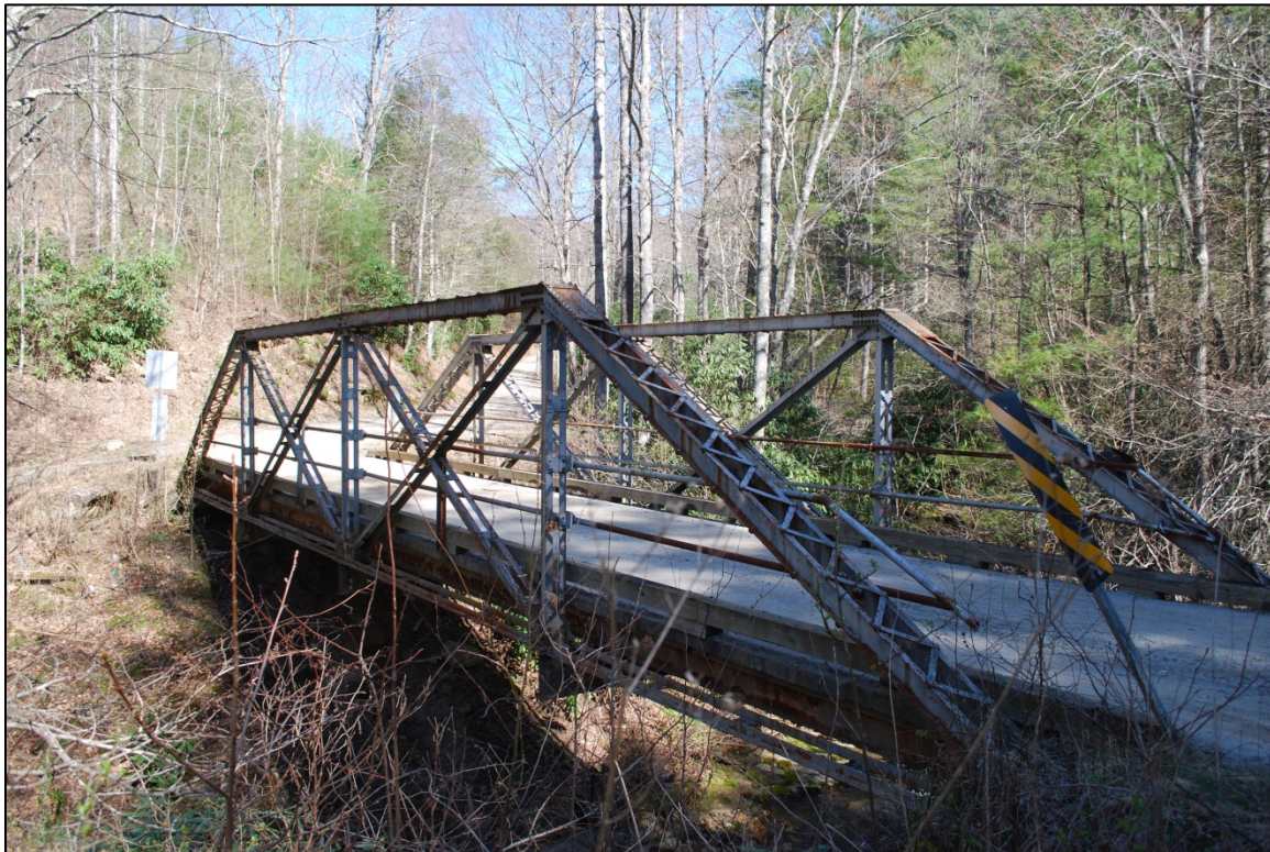
Figure 7: South elevation looking northwest.
